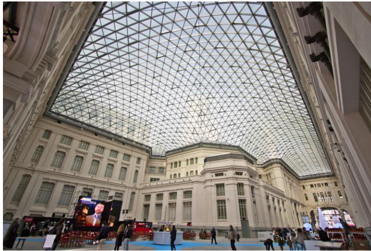
Figure 5: Courtyard of the town hall of Madrid. Notice the slight cable net under the gridshell. [Lanik]
