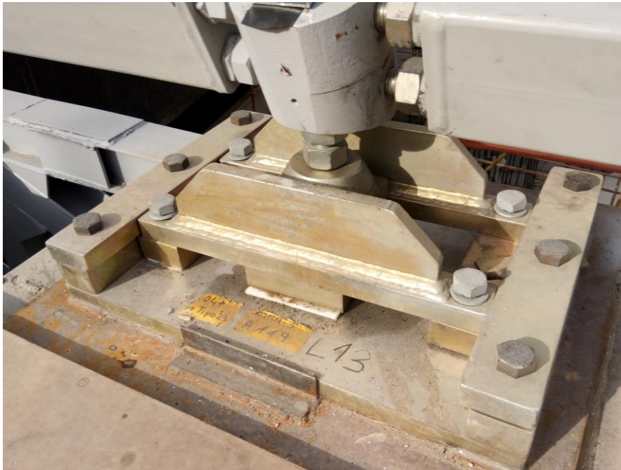
Figure 12: Special sliding support on site [Lanik]
