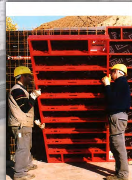
Domino Panel Formwork
