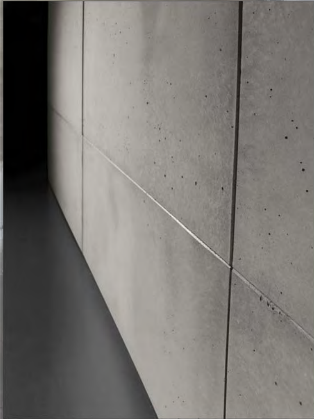
Smooth cement wall finish
