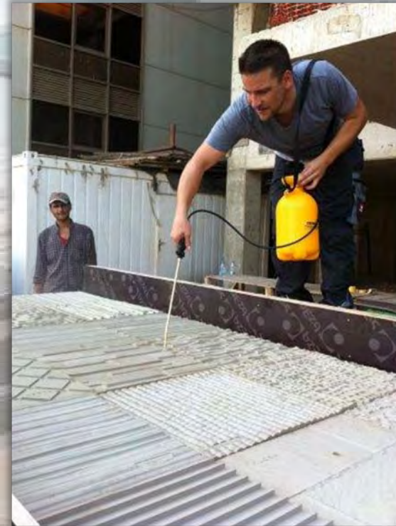
Step 2: Application of release agent on the molds
